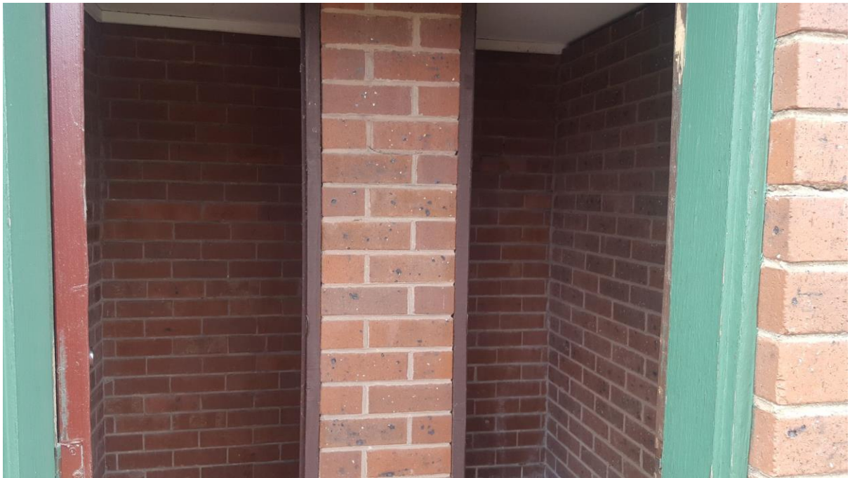
Rear Shed RHS
