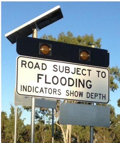
Figure 3 – Floodway warning signs with automated amber flashing warning lights
