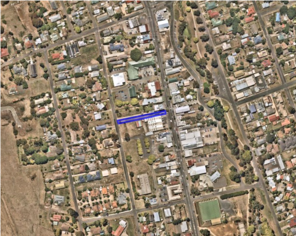
Figure 2 - NearMap Aerial Imagery of the surrounds (February 2021)
